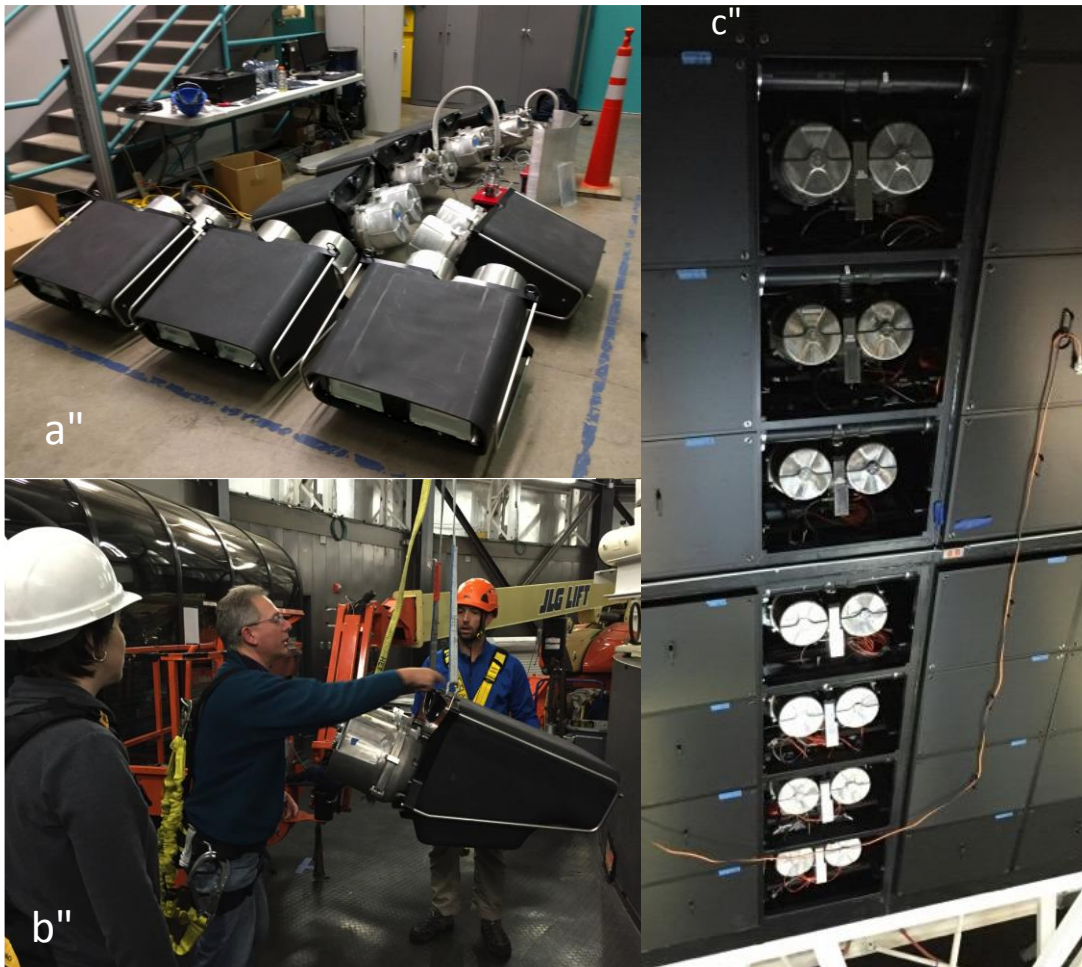
Figure 9: VIRUS spectrograph unit deployment; (a) 8 units staged for installation in HET receiving bay; (b) VIRUS unit rigged and balanced for lifting with HET dome crane; (c) 8 units installed in one of the VIRUS enclosures, prior to installation of enclosure covers.
